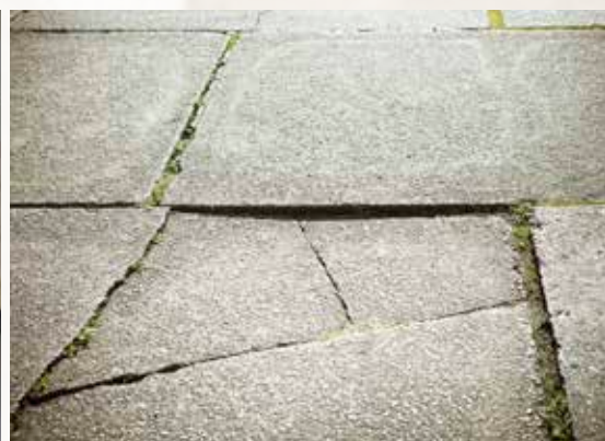
Concrete Lifting
