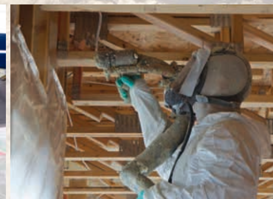
Rim and Band Joist
